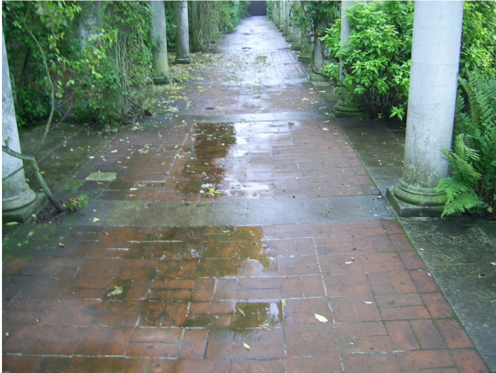
Photograph 4: Paviour pathway before replaying works
