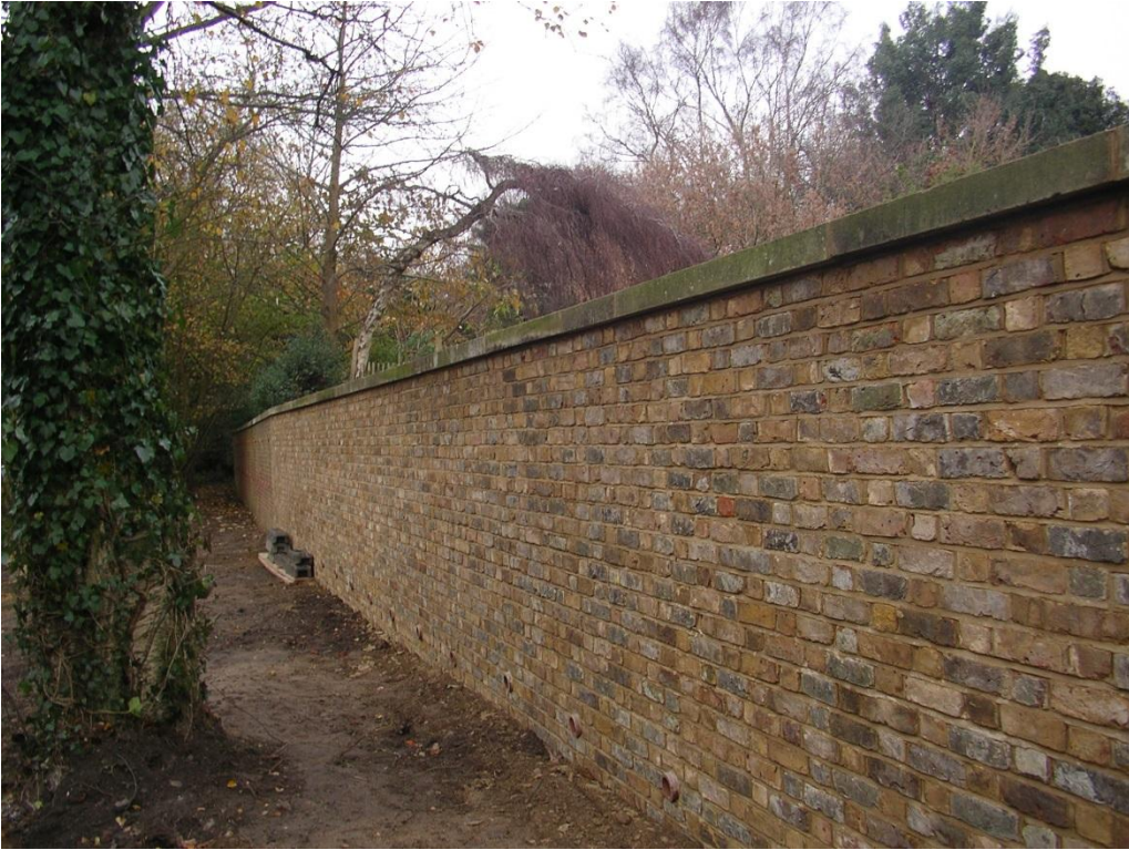
Photograph 7: Completed boundary wall repairs
